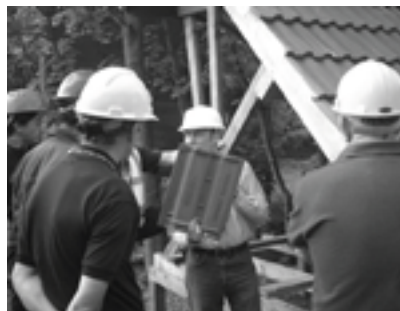
An explanation of roofing techniques during a PV training course
