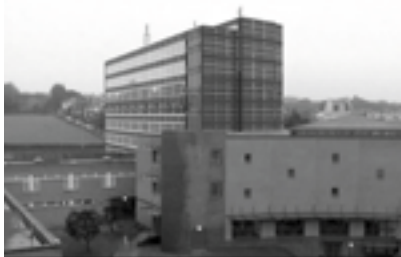
Proposed appearance of the refurbished tower block at Plymouth College of Further Education with PV facade
